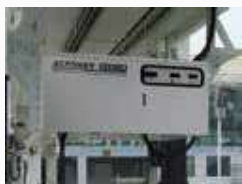
Airport Apron / Hangar
